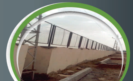
L&T phencing work at beawarpindwara expressway nh-14:
