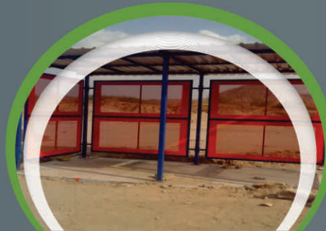
Bus shelter:- L & T n BPP projects (NH -14 EXPRESSWAYS)
