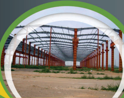
Large span peb structure:
