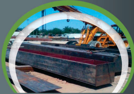
Heavy Fabrication work:
