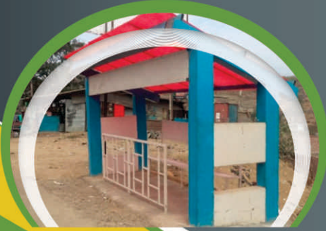
Bus Shelter:- (NH - 06 EXPRESSWAYS)
