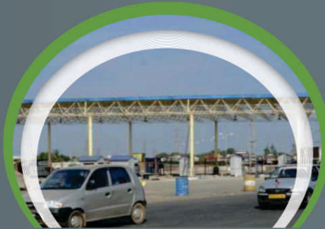
Space frame toll plaza canopy:
