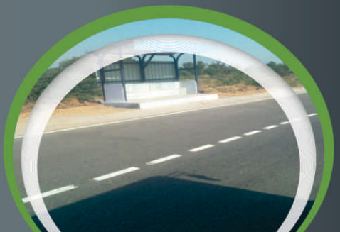
Bus shelter:- (NH - 08 EXPRESSWAY)
