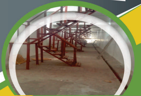
Toll Booth Canal work
