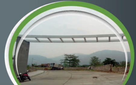
Site view Tower and Triple Storage Office
