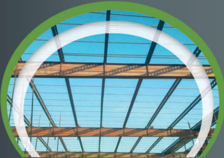
M.S. Structure work:
