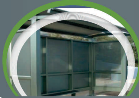
Bus Shelter Atyodhpur, Rajasthan
